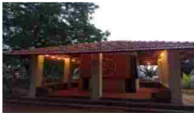
Low cost rammed earth building for coffee center
