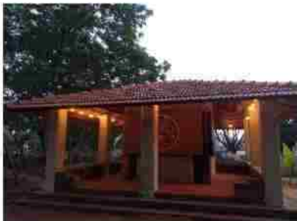
Low cost rammed earth building for coffee center
